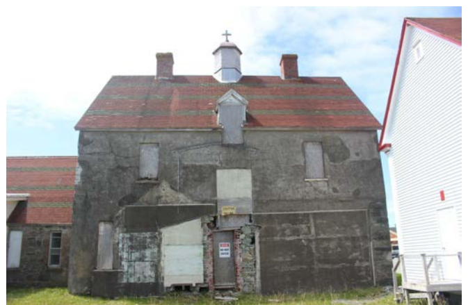
Fig. 7. Ghost marks on the rear of the convent indicate a number of former additions of various sizes and roof shapes. Source: Heritage NL.
