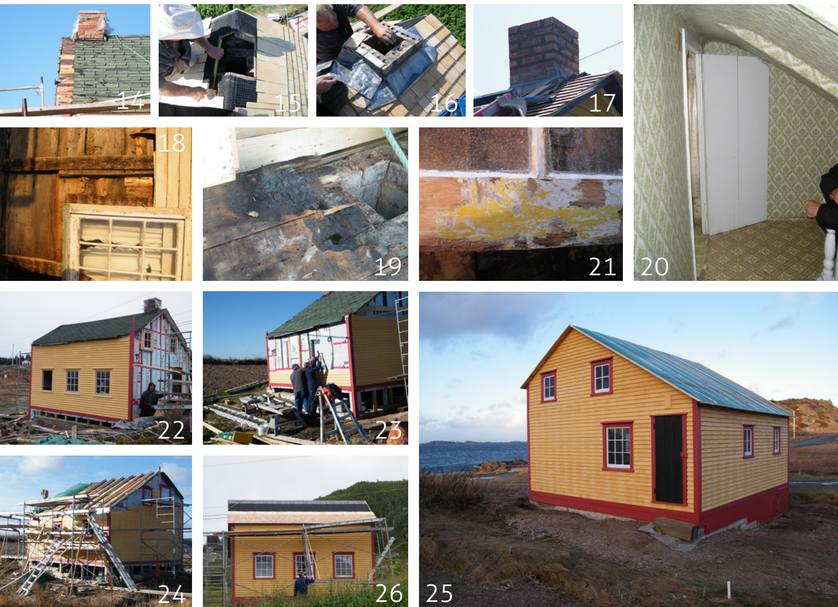
(14-17) The process of taking down and rebuilding the chimney; (18) stairhead window, uncovered during the restoration; (19) scorch marks on the boards around the chimney; (20) view of the upstairs landing; (21) scraped window sash, showing the earlier yellow ochre colouring; (22-24) exterior restoration work; (25) rear view, before roof shingles; (26) front roof, with wood shingles half installed; (27) exterior view, close to completion of project; (28) view of the completely restored Jenkins House Registered Heritage Structure.
