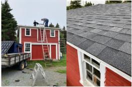
ROOF: Old shingles removed. Roof boards renailed. Rotted roof sheathing was replaced with new wood, and/or "Dutchman" repaired. The entire roof was reshingled. All fascia boards were rotted and replaced with new fascia boards.
