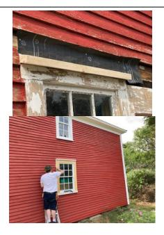
EAST SIDE (ocean facing side): Original clapboard was saved, re-nailed, scraped, caulked and painted. Windows restored.
