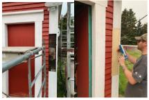
WEST SIDE: West facing side of the barn (treed side) required significant sheathing and corner rot replaced and or Dutchman repairs. All of the original barn interior framing was saved; the East barn sheathing/clapboard was restored and re-used.
