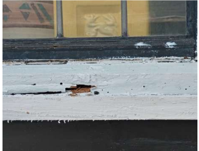
The window sill of window 1B2 has a small area of rot.
