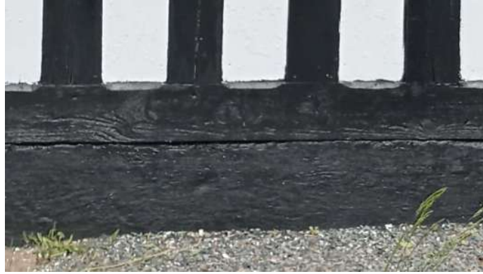
9 1/2 inch exposure on back elevation to the left of the addition
