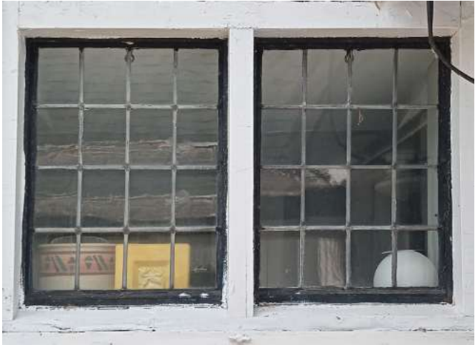
The window sill of window 1B2 has a small area of rot.
