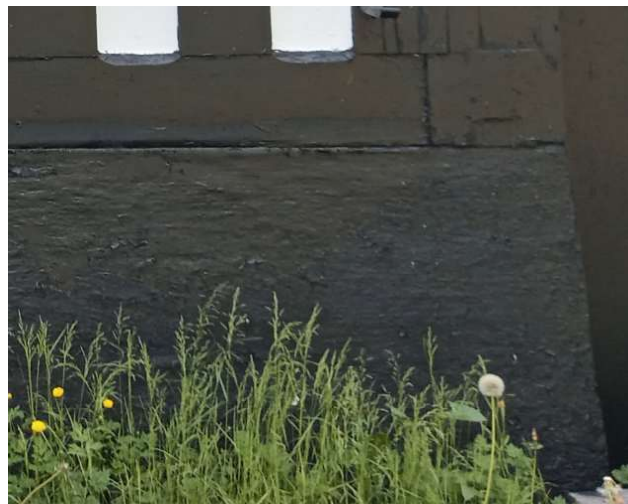
36 inch exposure on the back elevation to the right of the addition
