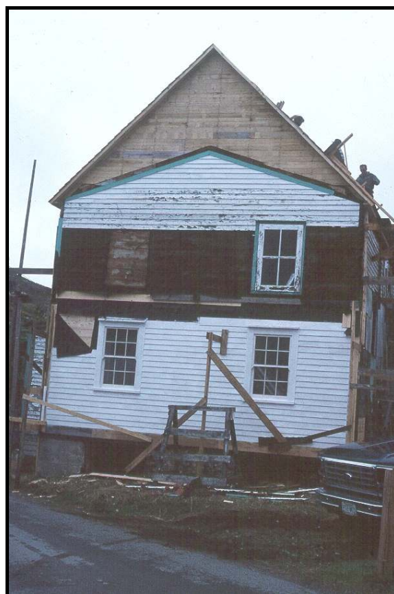
Original gabled roof under restoration
