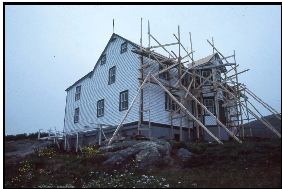
Bleak House under restoration.
