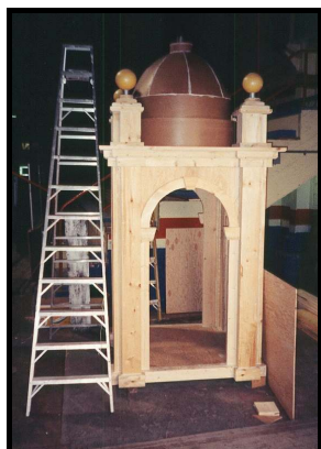
Rebuilding the cupola.
