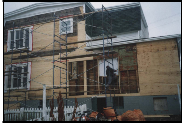
Lockyer/Swyers House under restoration.
