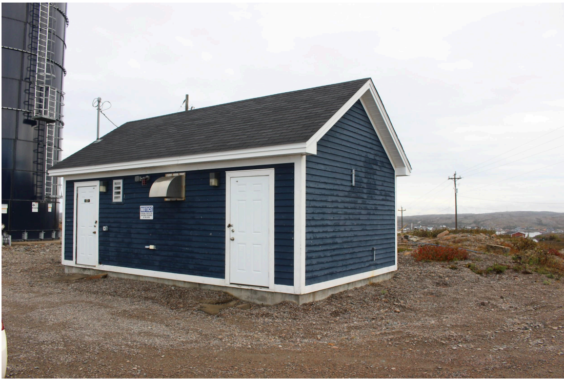
Joe Batt’s Arm Chlorine Building, 2023. Front and side facade. Photo by Juliet Lanphear.
