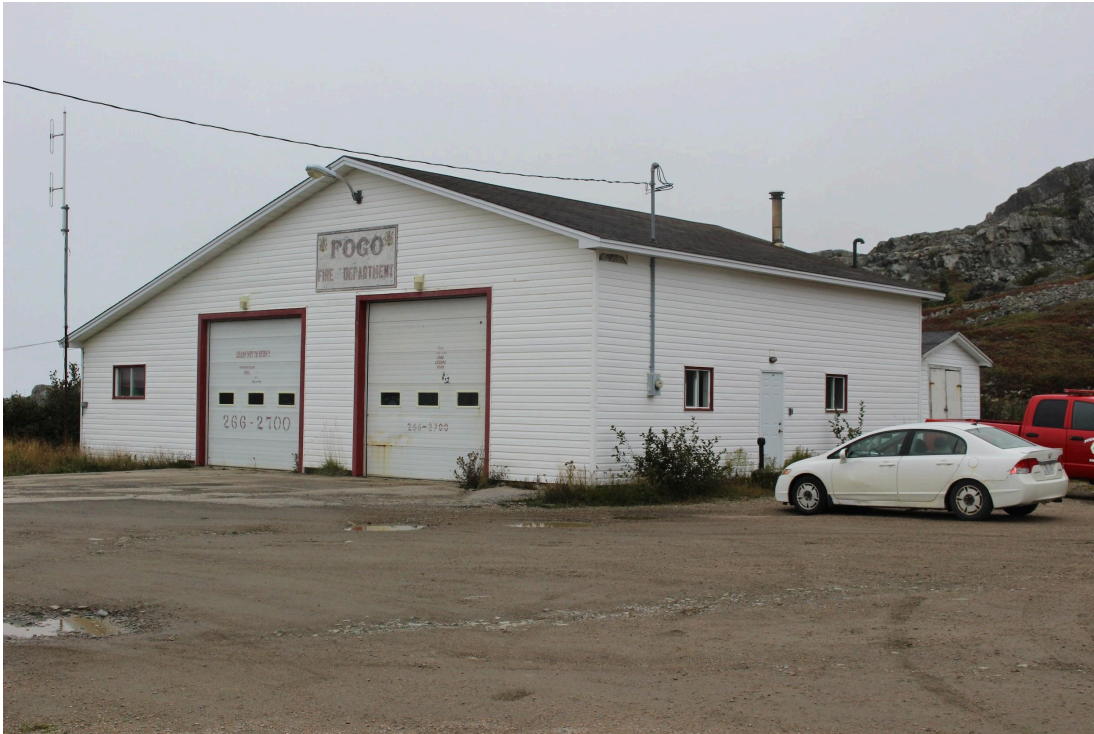
Fogo Fire Hall, 2023. Front and side facade. Photo by Juliet Lanphear.
