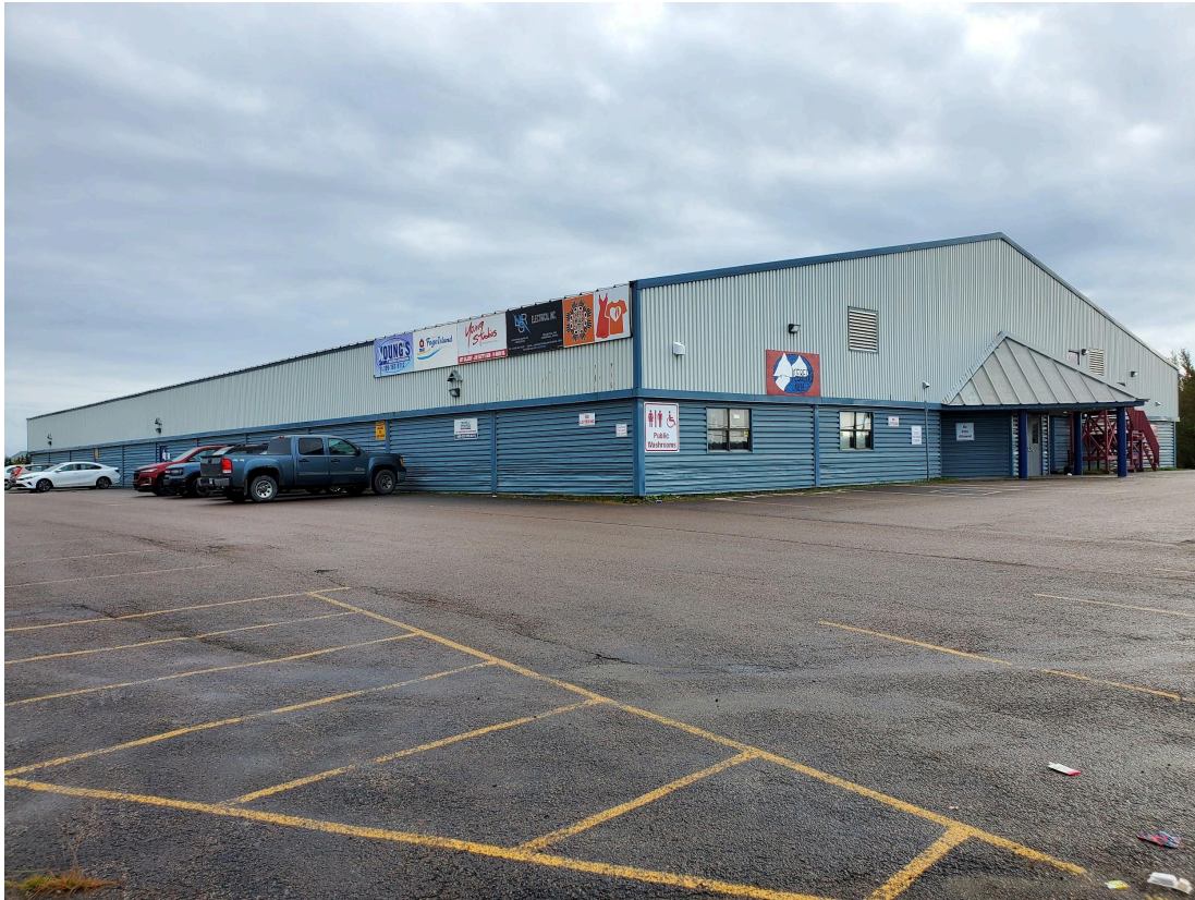
Stadium, 2023. Front and side facade. Photo by Juliet Lanphear.
