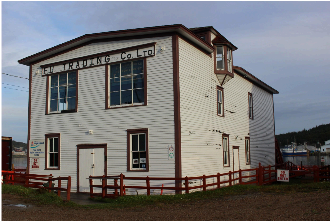
Marine Interpretation Center Building #1, the Fishermen's Union Trading Company Premises Registered Heritage Structure, 2023. Front and side facade.
