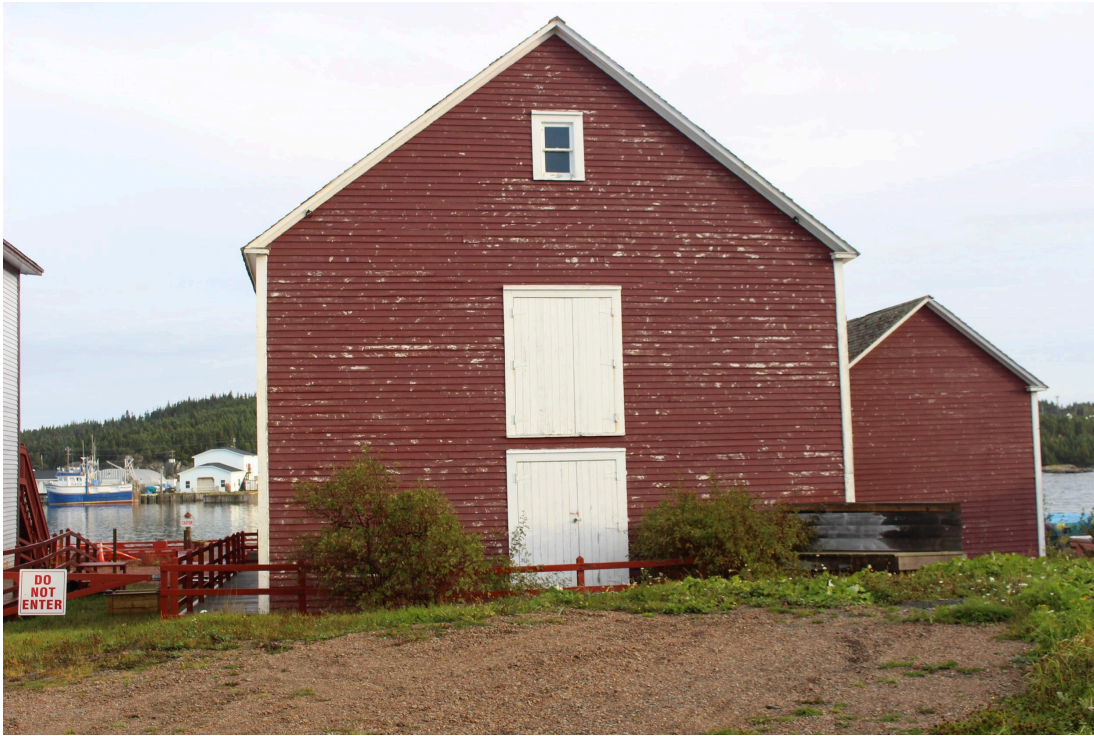
Marine Interpretation Center Building #2, Red Fish Store, 2023. Front facade. Photo by Juliet Lanphear.
