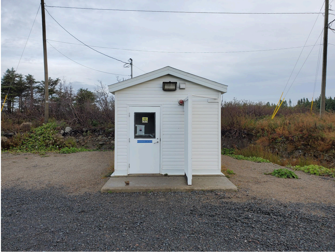
Seldom Chlorine Booster Station, 2023. Front Facade. Photo by Juliet Lanphear.
