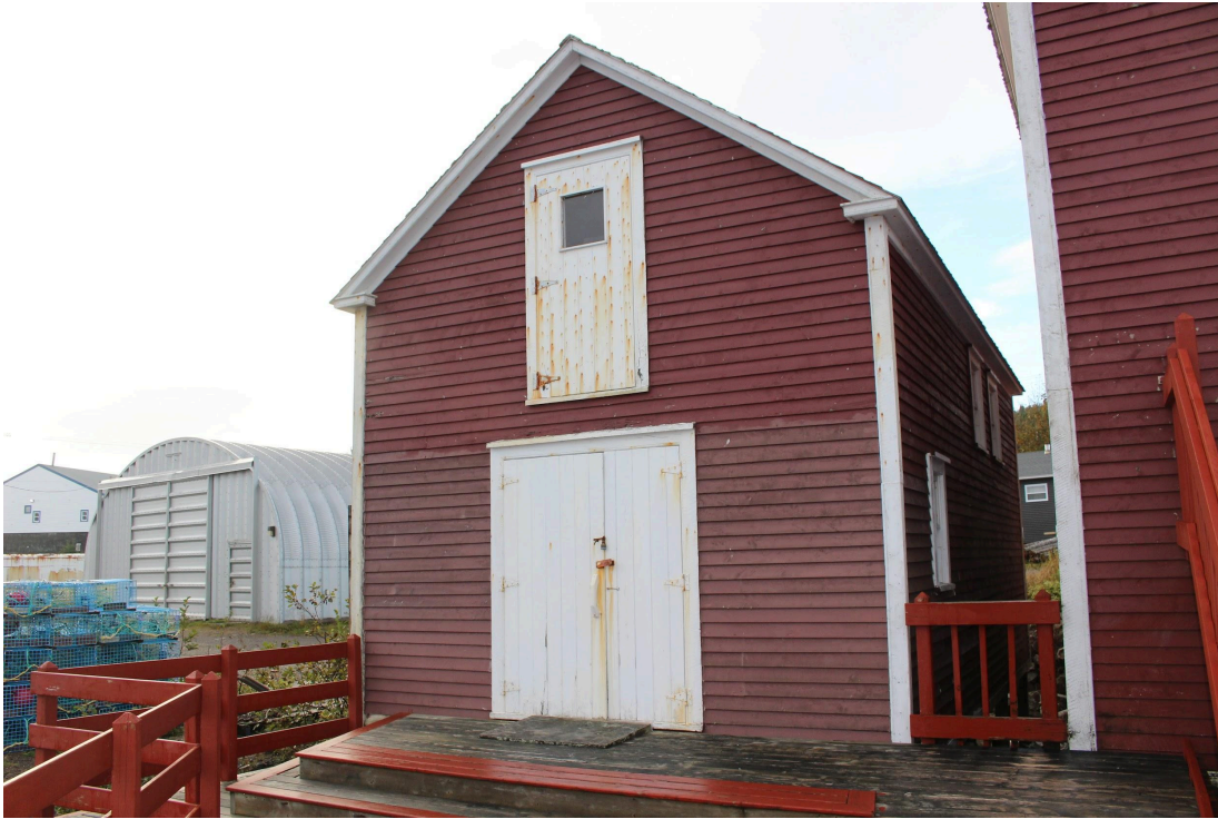
Marine Interpretation Center Building #3, Cod Liver Oil Factory, 2023. Front and side facade. Photo by Juliet Lanphear.
