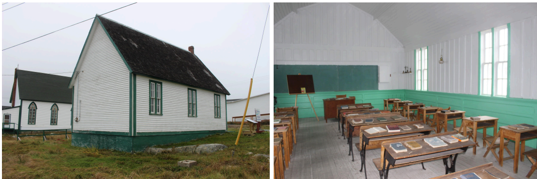
Old Roman Catholic Schoolhouse, 2023. (Above) front and side facade, (bottom left) back and side facade, and (bottom right) interior of the schoolhouse. Photos by Juliet Lanphear.
