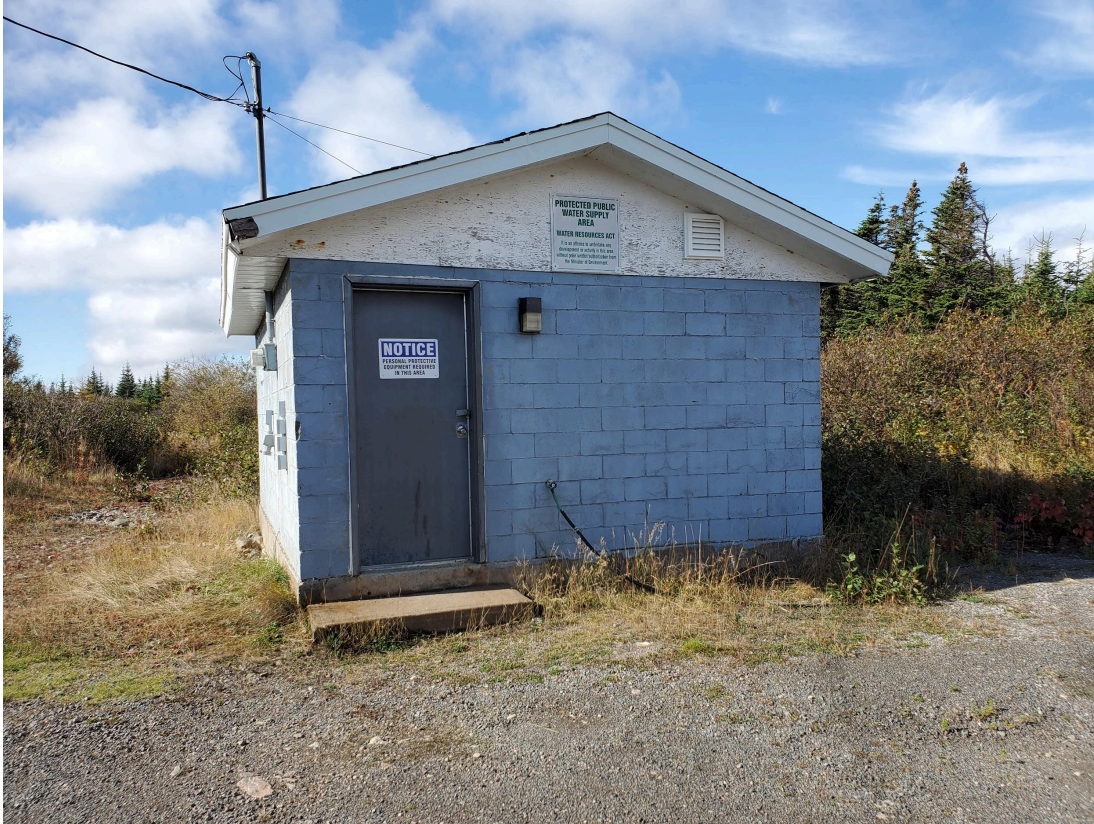
Tilting Pump House, 2023. Front Facade. Photo by Juliet Lanphear.
