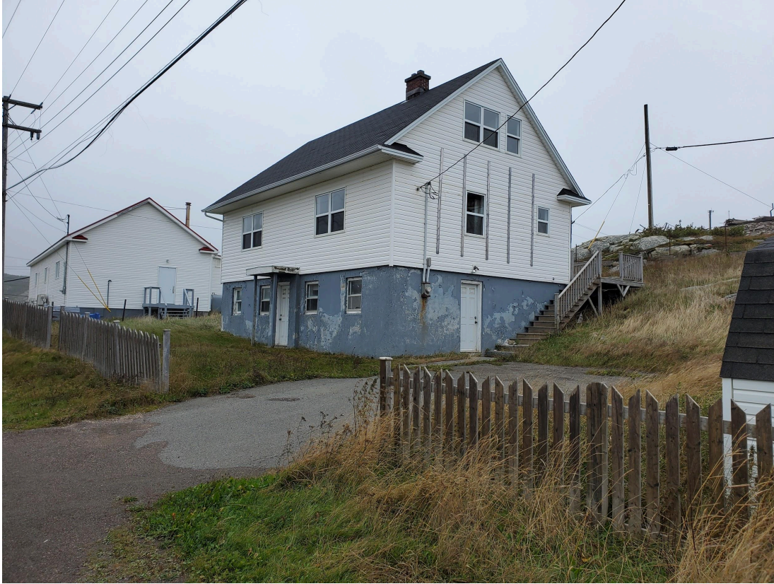
RCMP House, 2023. Front Facade. Photo by Juliet Lanphear.
