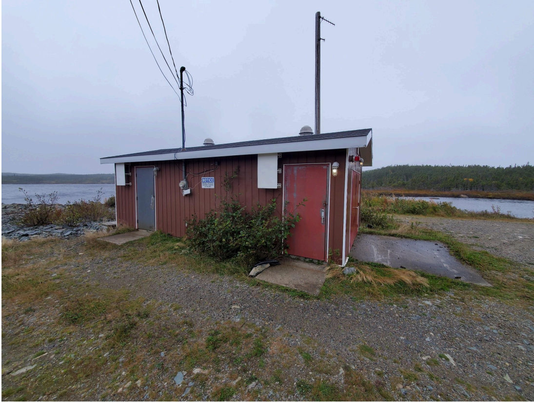
Fogo Water Chlorination Building, 2023. Side Facade. Photo by Juliet Lanphear.
