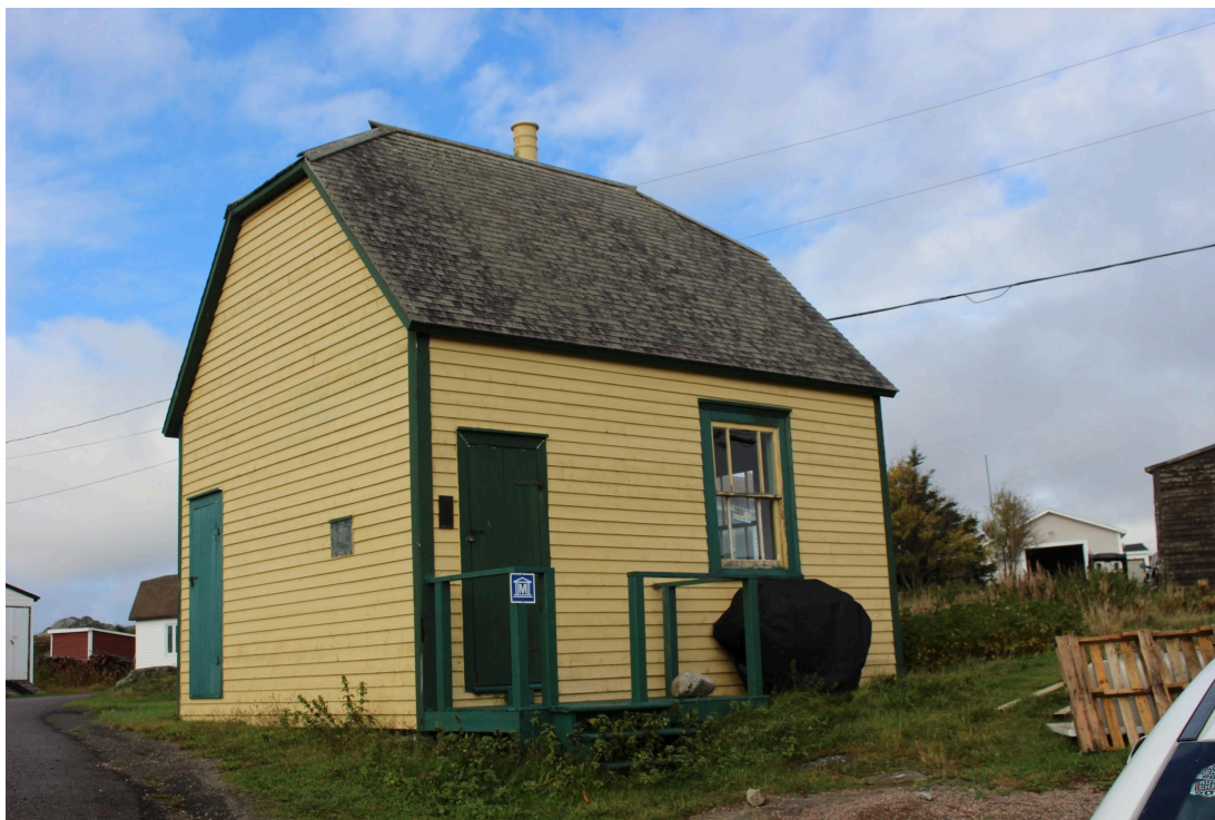
Old Post Office, 2023. Front and side facade. Photo by Juliet Lanphear.
