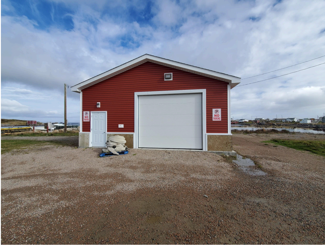
Tilting Fire Shed, 2023. Front facade. Photo by Juliet Lanphear.
