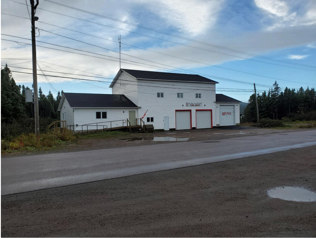
Seldom Fire Hall, 2023. Front Facade. Photo by Juliet Lanphear.
